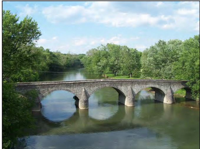
Photo 6: Wilson Bridge spanning Conococheague Creek
