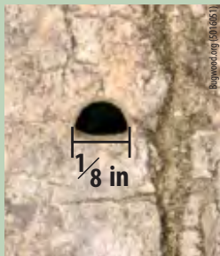
D-shaped exit holes
