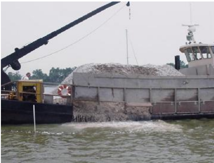
The Choptank Team used more than 100 tons of dredged oyster shell to create an oyster bar in Trappe Creek.
