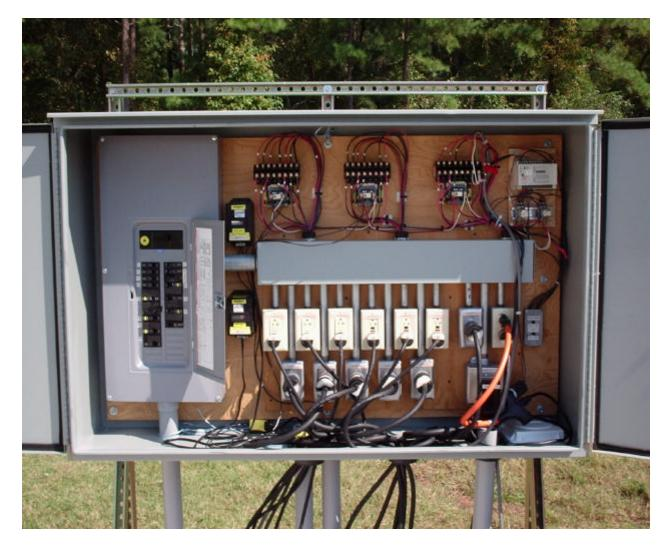
The electrical panel was constructed with the following features in order to achieve the split-pumping sequence:
