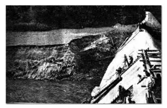
Figure 2. Flushing of accumulated sediment upstream of Bloede (ca 1920).
