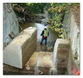
Figure 6. Sawcutting requires crane removal of large cut pieces.
