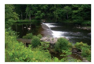
The McGoldrick Dam on the Ashuelot River was a six-foot high timber crib dam, built in 1828 and later capped with concrete. The dam diverted water into a power canal that supplied water to eight manufacturing facilities until 1950. The dam was removed in August 2001 to promote the restoration of a historic fishery.
