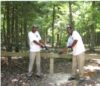
Our CJC team works on new parking area for group sites.
